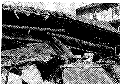
Photo 3 An example of old beam-to-column connections used in wood houses
