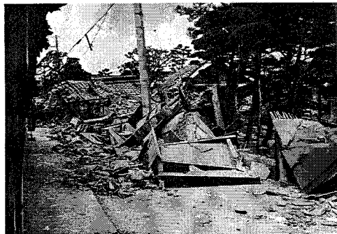
Photo 1 Collapse of wood houses roofed with heavy ceramic tiles
